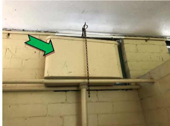
Photo 2. Interior, throughout, cistern – non asbestos-containing moulded fibre cement.
